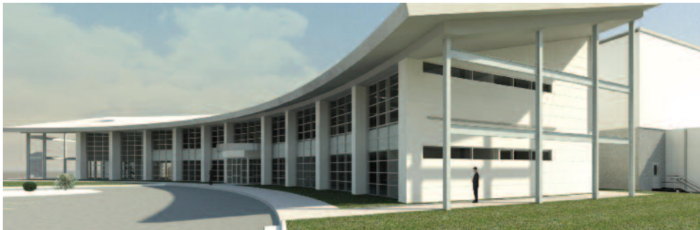
below: rendering of Siemens Wind Power's new nacelle assembly facility located in Hutchinson, Kan.
